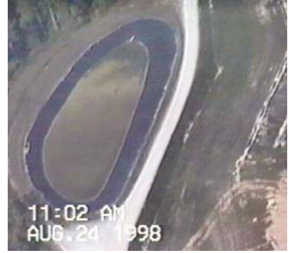
Kersey Valley leachate pond
