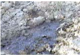
Kersey Valley Leachate spring.
